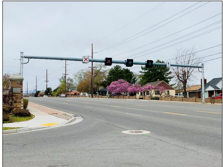
Figure 3-15. Overhead Gantry Example from Utah
