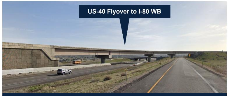
Elevated road or bridge that allows traffic to pass over existing roads or rail lines without having to stop or intersect at the same grade.
