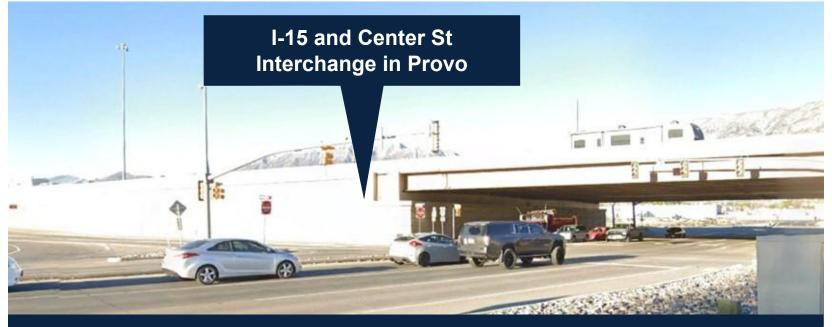
A tight diamond interchange features closely spaced, signalized intersections where freeway ramps meet the cross road to minimize the footprint.
