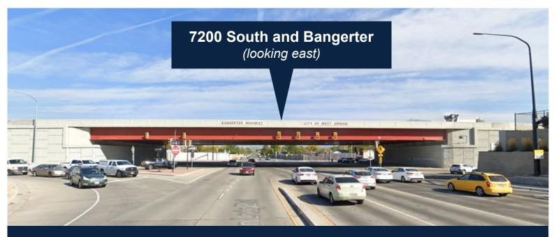
Streams of left-turning traffic do not cross, allowing the opposing left turns to occur at the same time.
